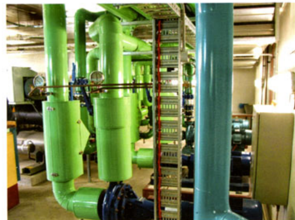
The completed pipes
